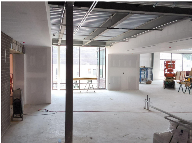
Addition looking south
