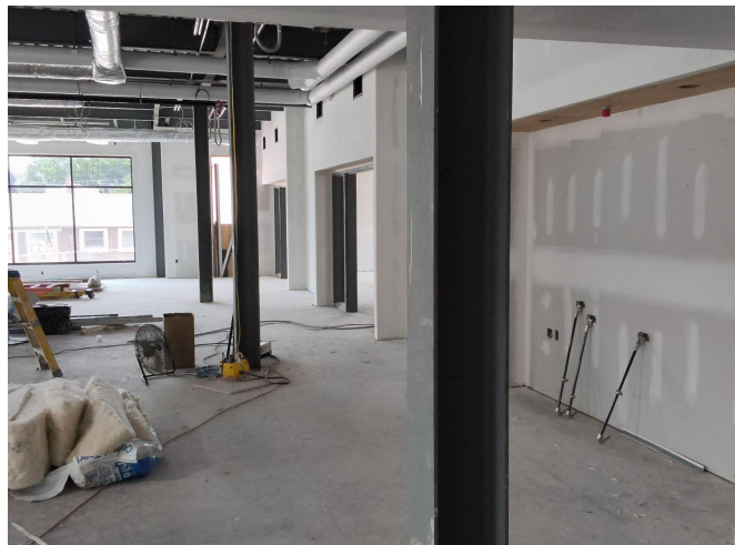
Addition looking west along community room
