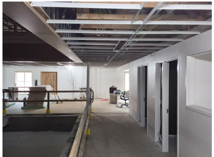
Original building - facing east
